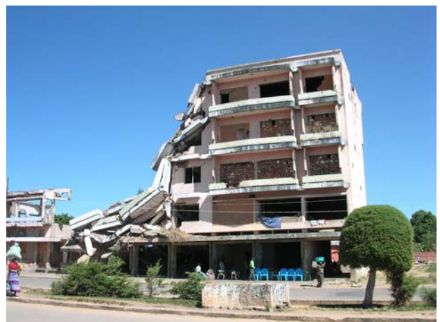
Fig. 5 Bombing during civil war in Angola destroyed much of the infrastructure
